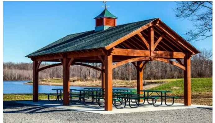
Figure 37: Custom Pavilion and Transportable Group Seating on Concrete Pad
