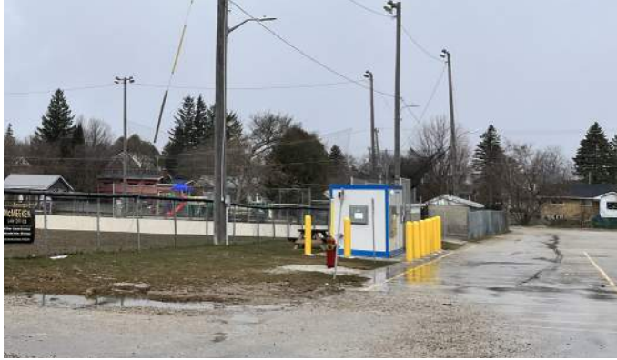
Figure 19: Bulk Water Filling and Dump Station
