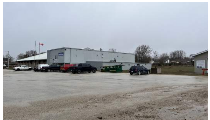
Figure 18: Non-organized Parking in front of Recreation Complex
